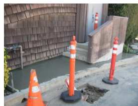
West side concrete repair
